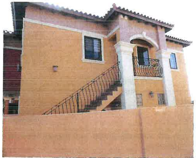
West side of the dwelling
