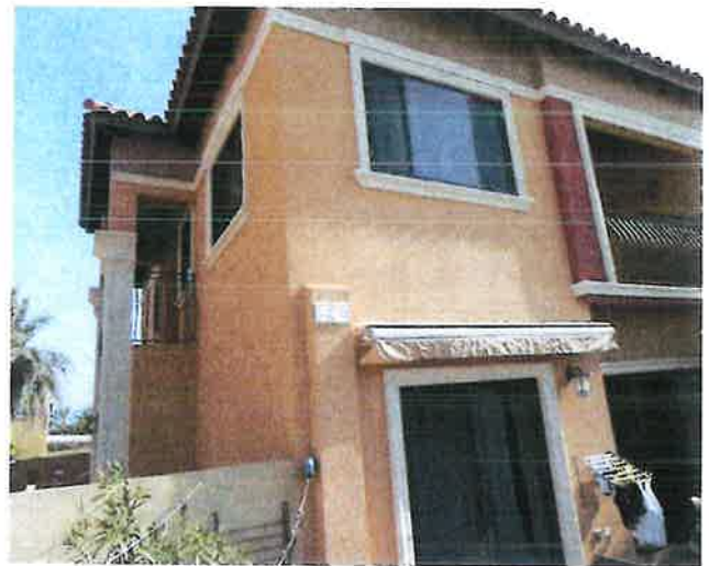
Rear side of the dwelling
